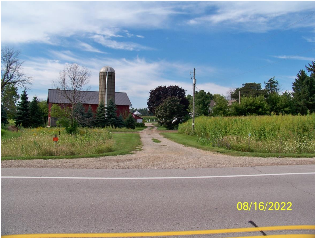
Overall view of the residence, barn and other buildings looking south.
